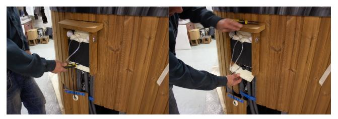
Use the box cutter knife set to 5cm depth and cut the insulation carefully, as shown.
