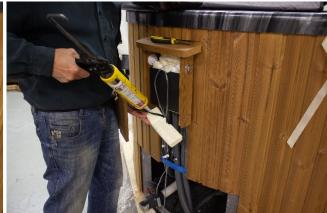
Insert the new control through the hole as well as the retaining nut. Here also apply silicone to the cut in the insulation.
