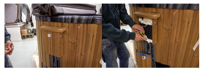
Remove the 4 screws from the control box.
